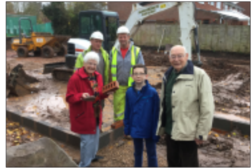
Community project - Niall Meades, Anne Kirby and Michael Kirby with contractors on the site of St Chad's Community Centre. (s)
